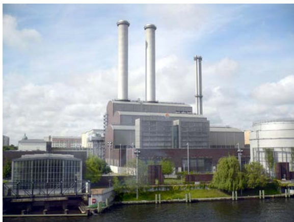
Combined Heat/ Power Plant(CHP), Berlin-Mitte
