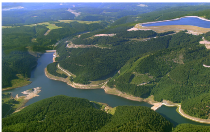
Hydro Pumped Storage, Germany
