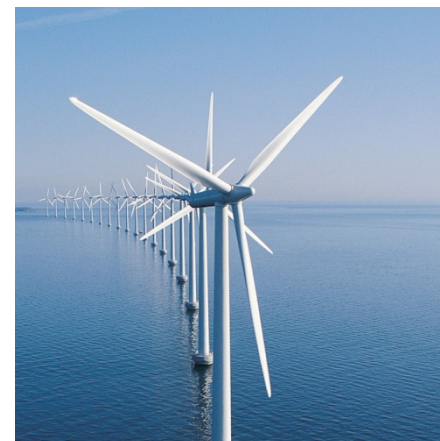
Offshore Wind Farm, Denmark
